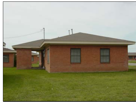
800 Getzendaner Street, rear facade, erected 1951
