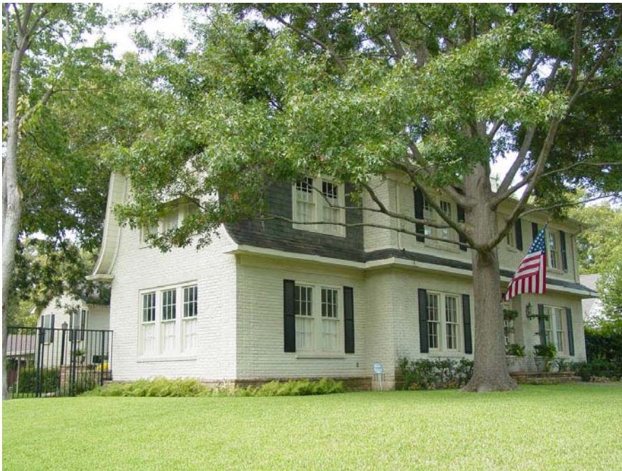
Sycamore Street. Dutch Colonial Revival dwelling.
