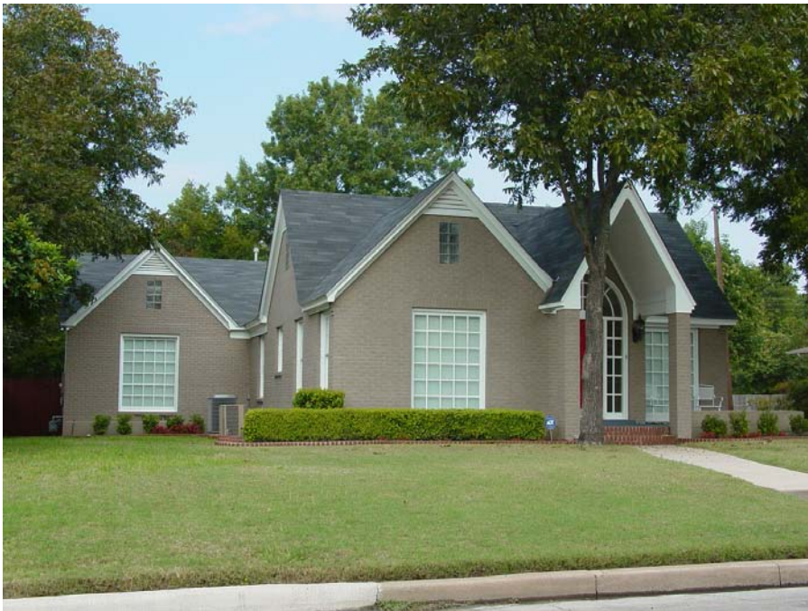
Dwelling, Harbin Street. Showing porch alteration.
