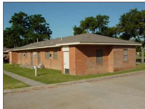
208 Patrick Street, rear facade, erected in 1951.
