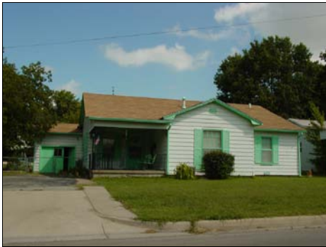
105 Olive Street, erected c. 1955
