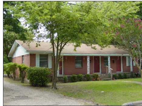
206 Olive Street, erected c. 1955
