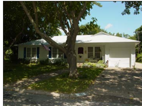
101 Wilmington Ave., erected c.
